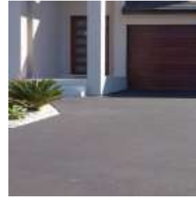
Coloured Concrete driveway
